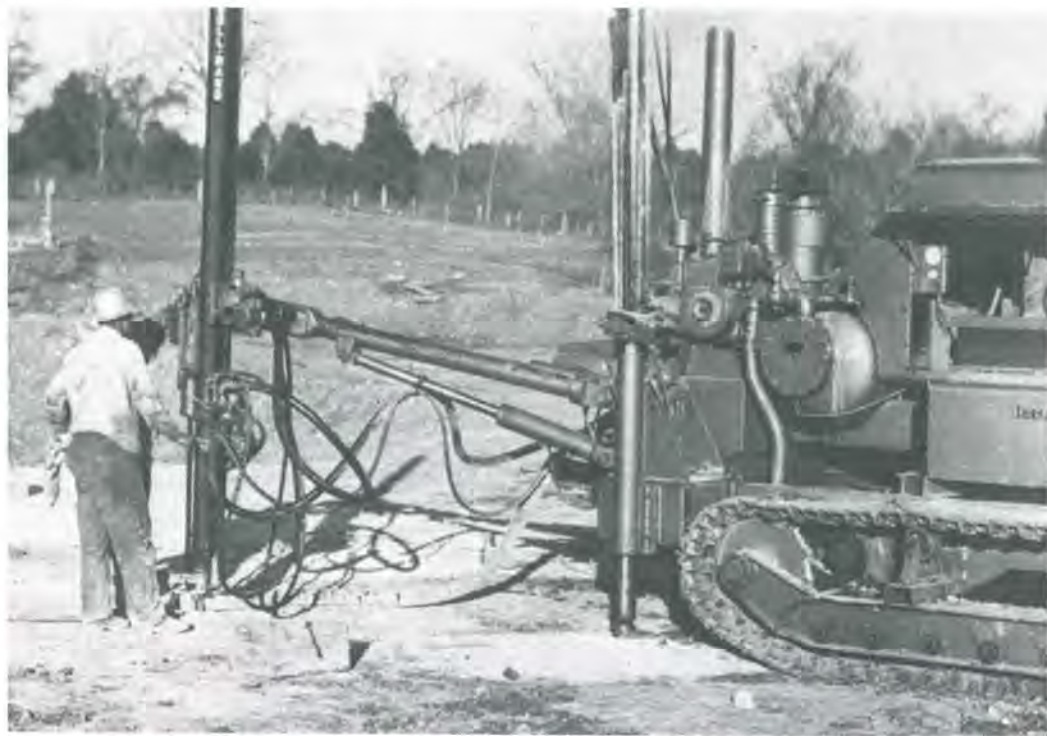
Workers use an Ingersoll-Rand Drillmaster at the quarry site built to provide material for the Gallatin Steam Plant in 1954. Note the early use of hard hats, well before government agencies required them.
