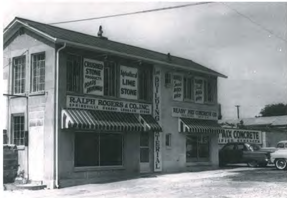
Ralph insisted that his companies always look neat and would occasionally shut a quarry down if it wasn't neat enough for him. On photo day, at least, this operation outside Bedford, Indiana, likely passed muster.
