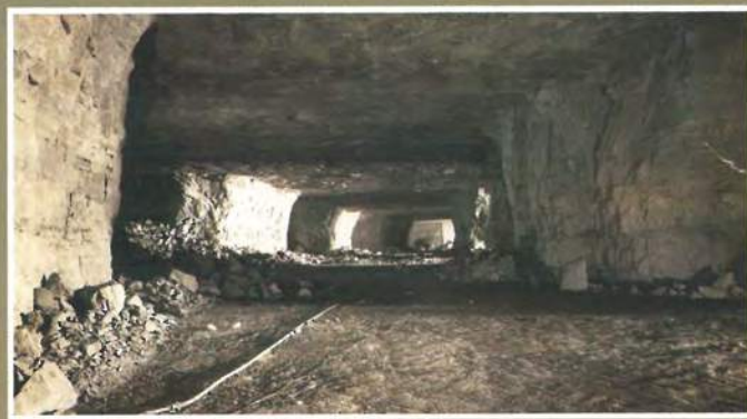
In the 1940s, trucks at the Louisville mines were loaded underground. The miles of corridors always caused a safety concern in the mines, sending superintendent Ora Brown into the tunnels nightly to listen for cracking and popping. These days, conveyors bring the crushed stone to the surface where it's sorted. Photo courtesy of John W. Salsman, Lewisburg, Tennessee.
