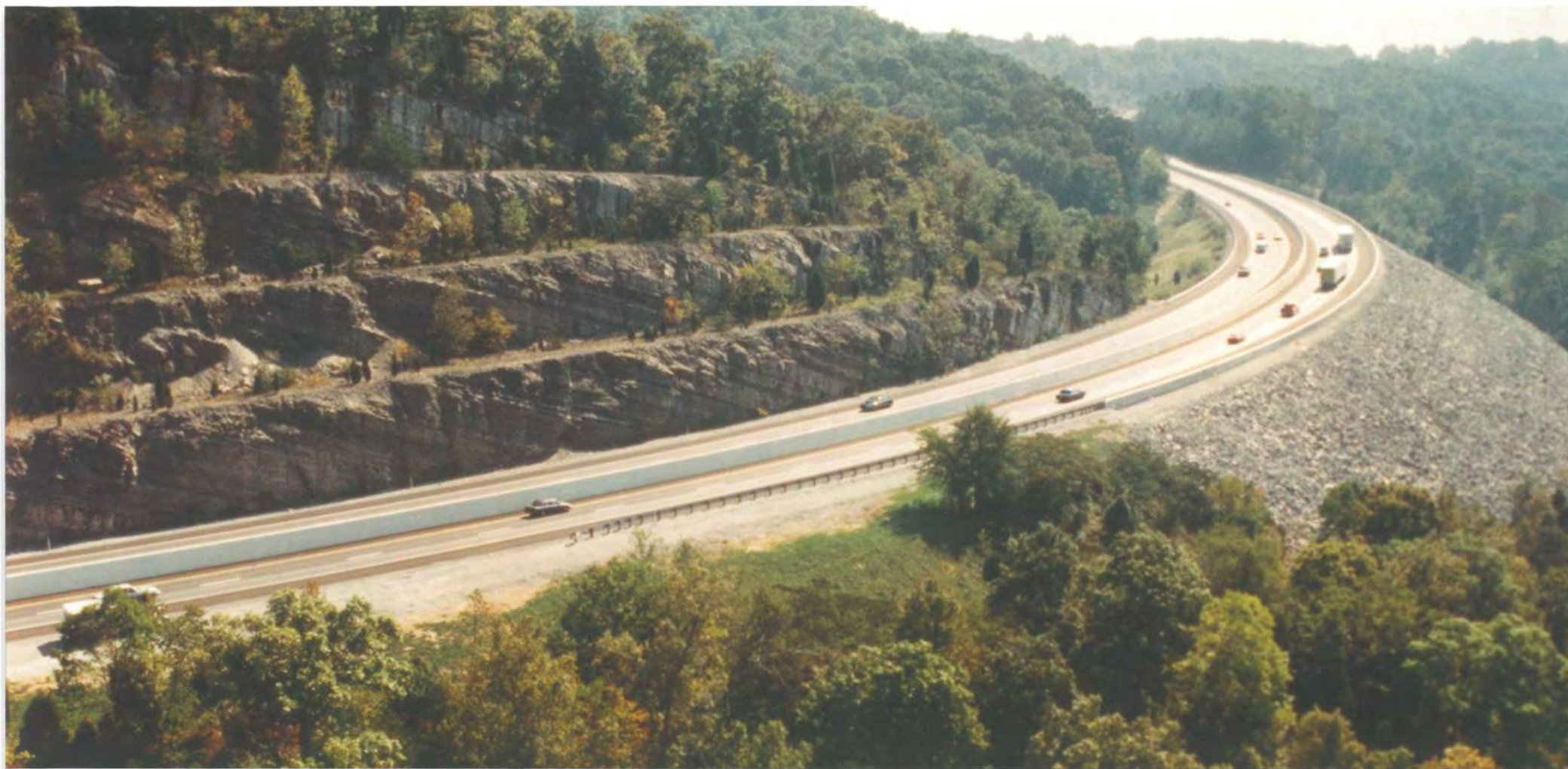
Interstate 75 in east Tennessee is an example of Rogers' interstate construction.
